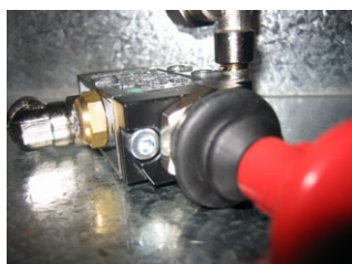
Valves with fittings and silencer
